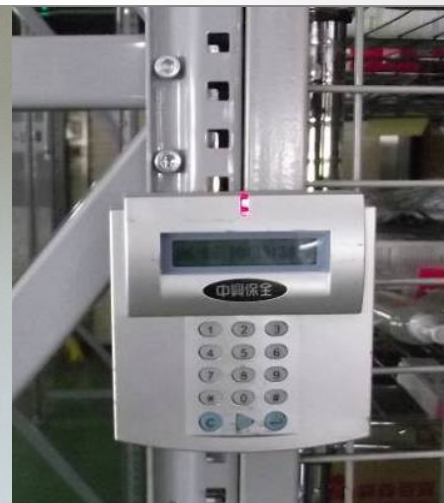
RFID Protected Doors
